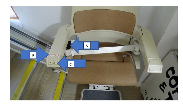
5. The stair lift is now ready for action. The passenger can control the chair using the direction buttons (C). Should they not be able to, there are override buttons adjacent to the chair lift at both ends of the staircase.
